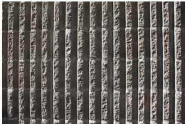
**Figure 9 – Fluted Concrete Block Wall Texture**
