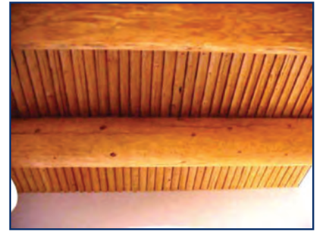
Viga and Latilla Construction
