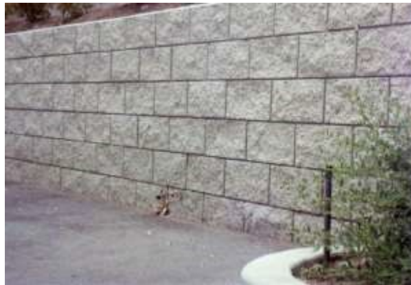
Figure 8. Split Face Block Wall
