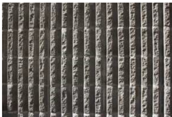
Figure 9. Fluted Concrete Block Wall Texture
