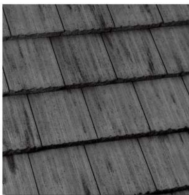
Roof: 303 Sierra Madre- Ponderosa Mfr: Eagle Roofing
