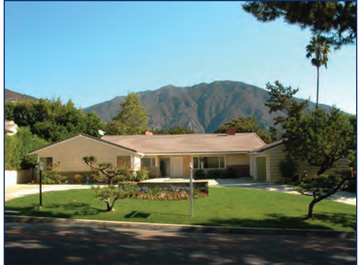
Low pitched roof and side entry garage
