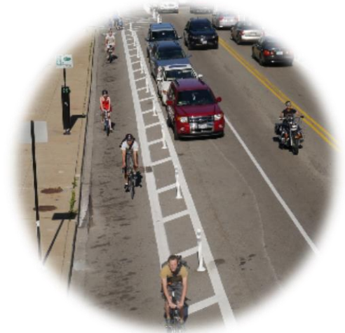
Typical Protected Bicycle Lane: Lake Street, Chicago, IL (Green Lane Project of PeopleForBikes at www.peopleforbikes.org )
