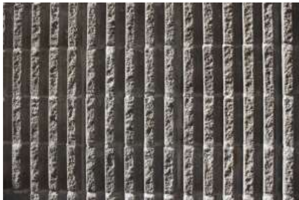
Figure 9 – Fluted Concrete Block Wall Texture
