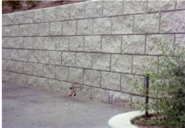
Figure 8 – Split Face Block Wall
