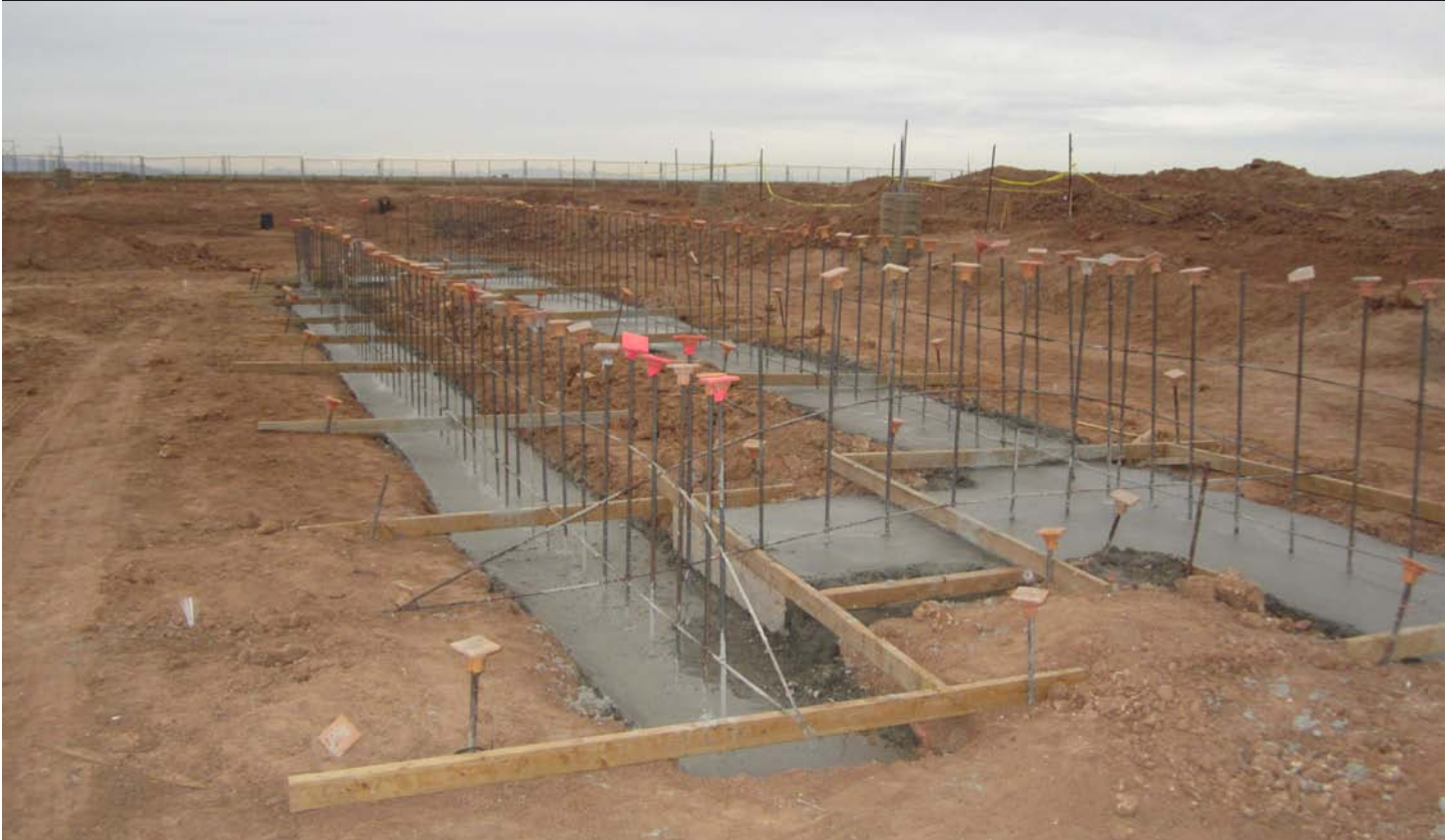
Concrete Footings for Retaining Wall on West Side of City Hall
