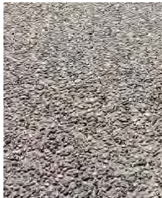
CONCRETE EXPOSED AGGREGATE FINISH
