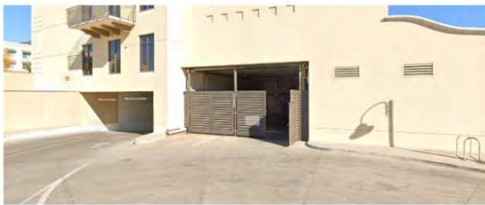
Under Building- Ventilated
