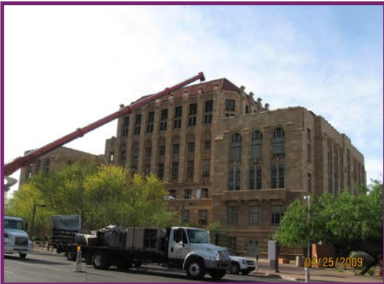
Maricopa County JOC - Old Courthouse HVAC Upgrades
