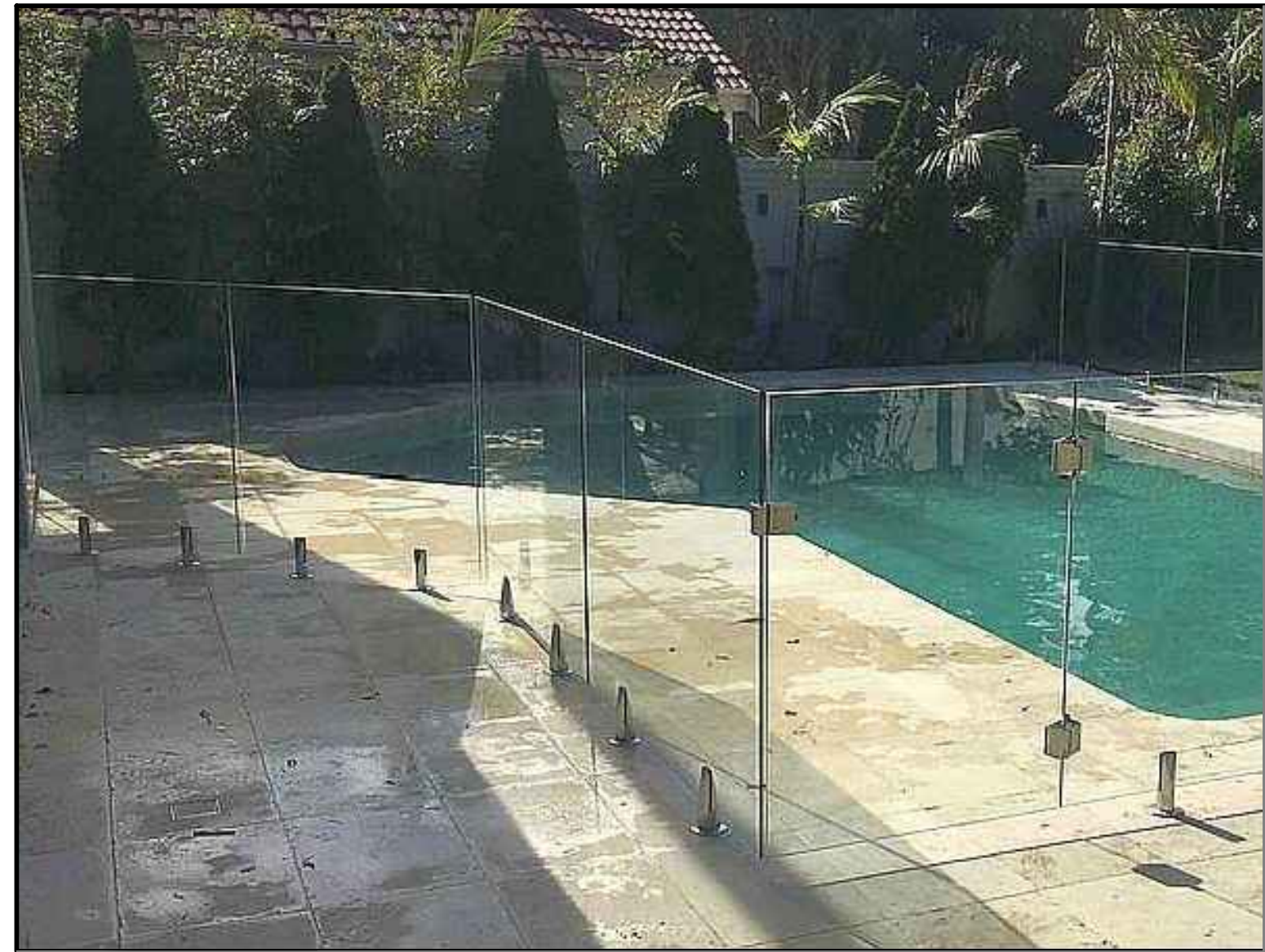
05 POOL BARRIER. 5' TALL GLASS BARRIER
