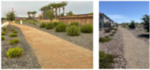
10' COMPACTED 50/50 SAND VEHICULAR MAINTENANCE AND PEDESTRIAN TRAIL
