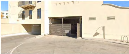
Under Building- Ventilated
