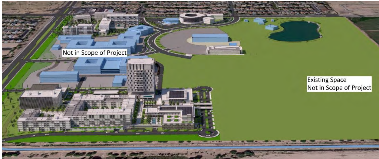
Overview of D3 PAD Project
