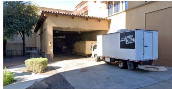
Adjacent to Building- Ventilated
