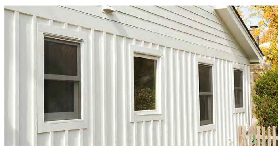
HARDIE BOARD VERTICAL BOARD AND BATTEN SIDING
