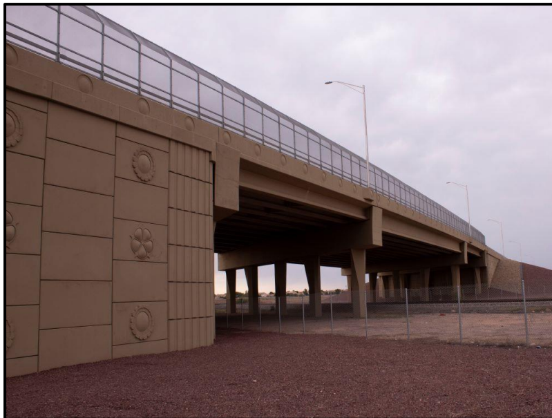
Figure 22: Freeway Overpass Art
