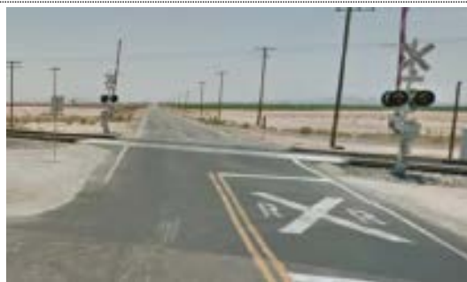
From the intersection of Maricopa-Casa Grande Hwy looking south on Anderson Rd across UPRR
