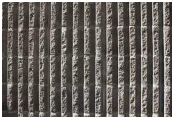
Figure 9. Fluted Concrete Block Wall Texture
