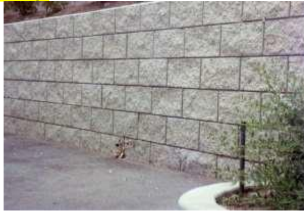
Figure 8. Split Face Block Wall
