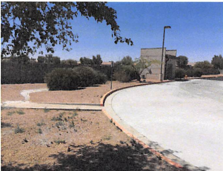
City of Maricopa Fire Station 574
