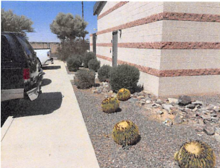
City of Maricopa Fire Station 571
