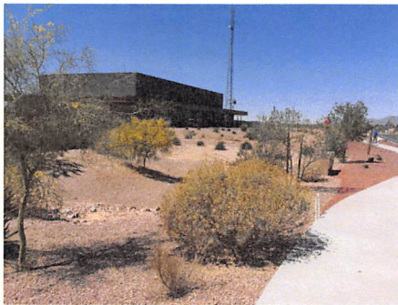
City of Maricopa Fleet Maintenance Building
