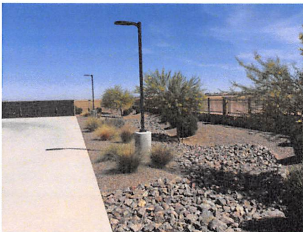
City of Maricopa Fire Station 572
