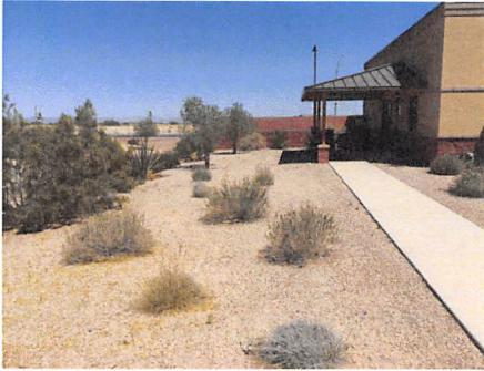
City of Maricopa Fire Station 575
