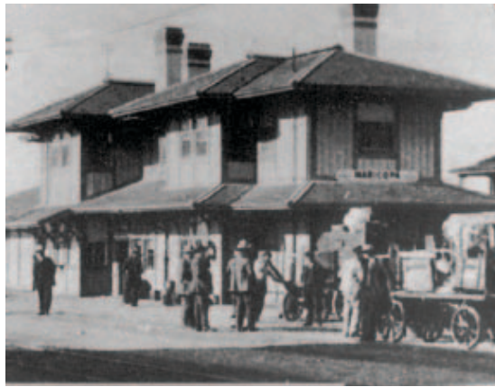
(Maricopa Railroad Station)
