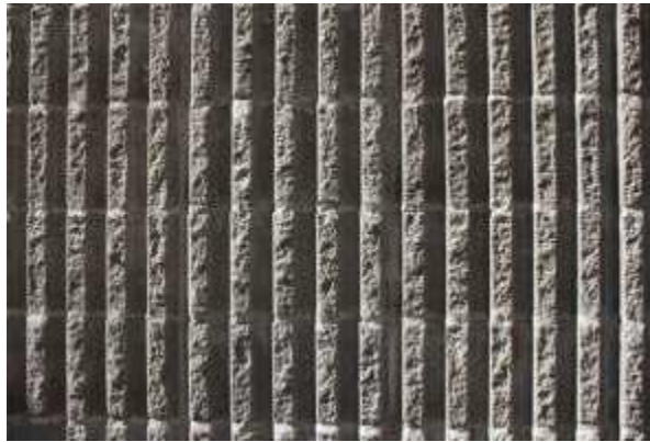
Figure 9. Fluted Concrete Block Wall Texture
