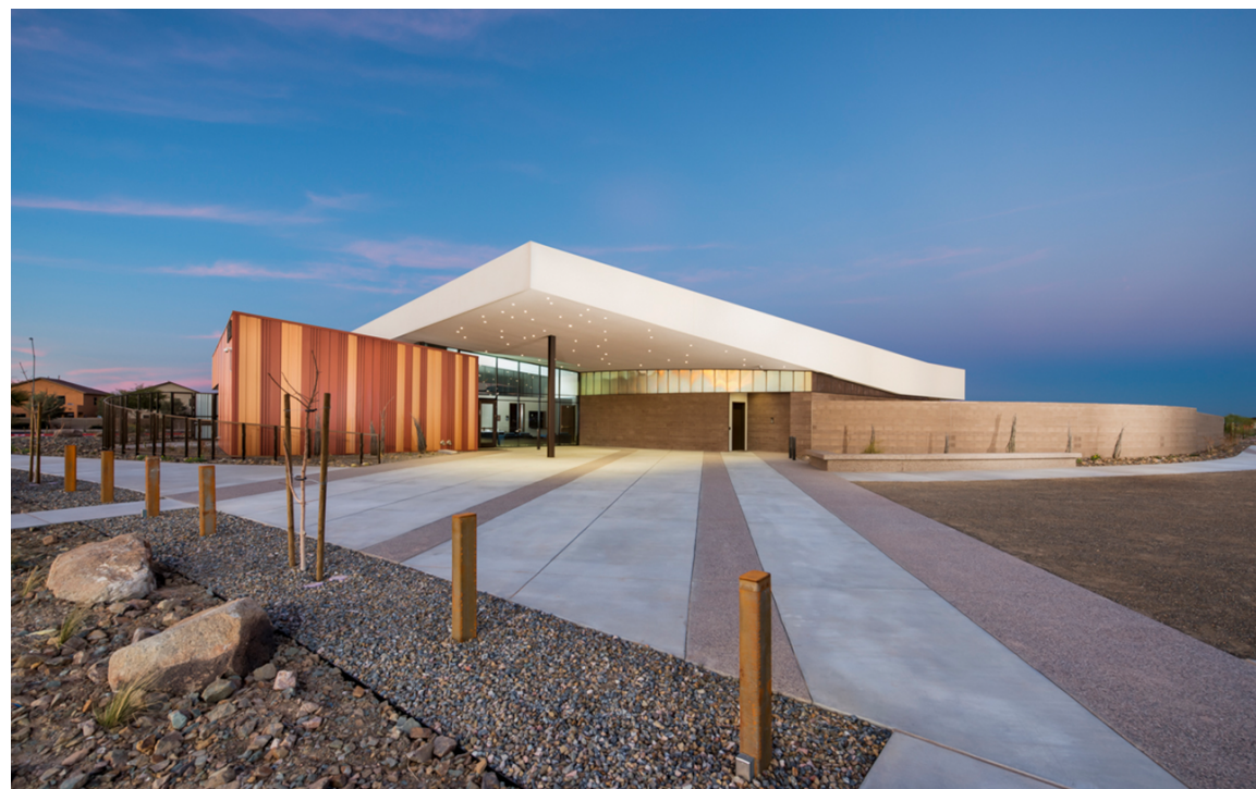
EXISTING PD SUBSTATION COLOR AND MATERIALS
